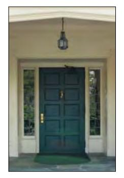
Follow and adapt successful historic patterns. When repairing or replacing elements in the front entryway, match the original in sizes and scale. Retain as much original historic material as possible. Slope exterior surfaces away from the entry door. Only where deep shelter is provided can the entry material be flush with the door threshold, as in the example above.
