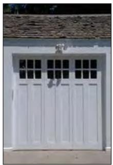
Garage doors should be compatible with the character or the accessory building. Wood hinged doors are preferable. In cases where replacement is necessary, replace to imitate the original structure. Here the window size has changed, and the door is an overhead-swing model, while still *matching the historic character.*
