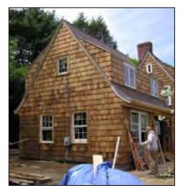
Design additions that use building forms similar to those of the historic building. In this example, the roof shapes and lines of the original building are used on the addition. Also, the addition is lower in height and smaller in scale that the original.
