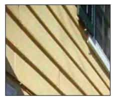
Replicate original clapboard siding in exposure, detail and dimension. Install replacement clapboards of clear grade, solid material, and of a board length no less than 48 inches.
