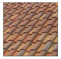
Replace damaged historic terra cotta roofing with new tiles that match original in material, color, decorative patterns and style.
