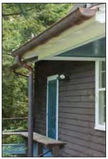
Downspouts should be the same material as the gutters. Copper should remain natural, not painted. Copper and stainless steel have the longest useful life, as much as 100 years or more. Galvanized steel can last for 50 years or more with proper care, and its lifetime can be longer if painted. *New non-lead bearing coatings are* available to substitute for such historic materials as lead-coated copper, or lead/tin flashing and solders.
