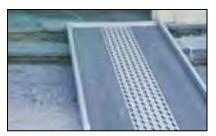
*Where possible, changes to historic* entryways should be reversible. For example, a handicapped access ramp is installed in a manner that does not alter the original design of the steps and portico floor.
