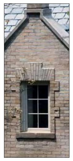
Before starting an historic masonry project, identify masonry features that are key to the building's overall historic character. Document masonry unit type and size, masonry color, bonding patterns, mortar joint type and size, and coatings.
