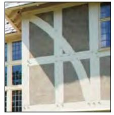
Use brick masonry fill, nogging, wattle and dawb, plaster or stucco fill with half timber construction. Nontraditional resin-based stuccos are not allowed for any repairs, restorations, additions or new construction.
