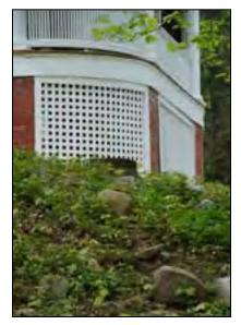
Retain and preserve original lattice. For replacement, retain original scale and proportions. Install lattice in framed sections with casings a minimum of 3.5"). Orient lattice vertically and horizontally unless there is strong evidence of an original diagonal arrangement.
