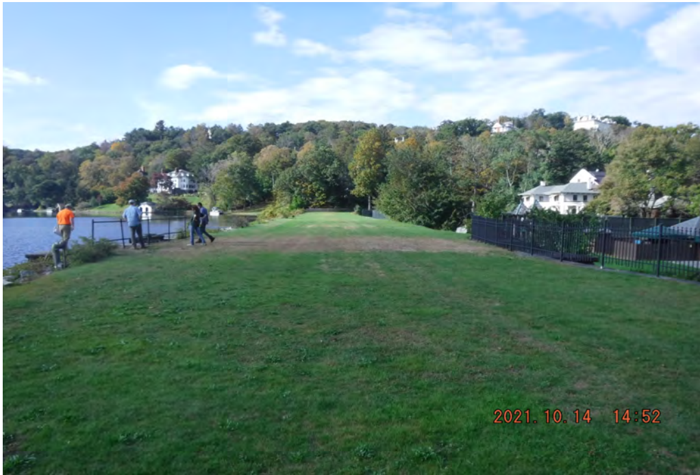
Photo 5 Dam ID# 196-0354 Tuxedo Lake Dam 10/14/2021 Dam crest View looking left from right end of dam
