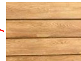
CUSTOM FRONT DOOR & UNDERSIDE OF EAVE SIBERIAN LARCH WOOD NATURAL CLEAR COAT
