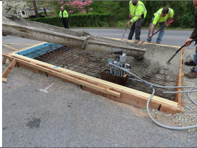
Foundation forms and reinforcement in place as concrete is poured
