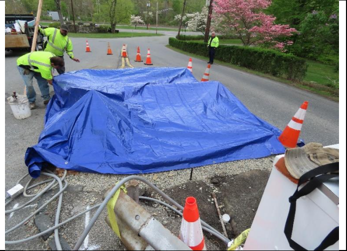
Finished concrete foundation slab protected from rain with tarp
