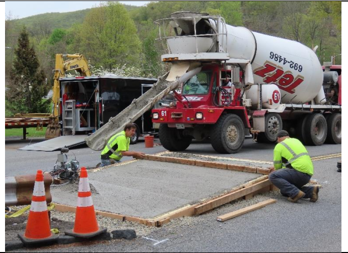
Concrete is leveled with screed
