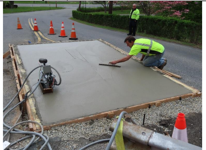
Final troweling to complete concrete foundation
