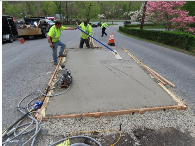
Concrete finished surface is leveled with float
