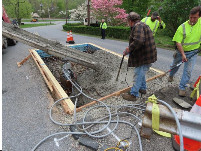
Concrete is moved through reinforcement with vibrator and rakes
