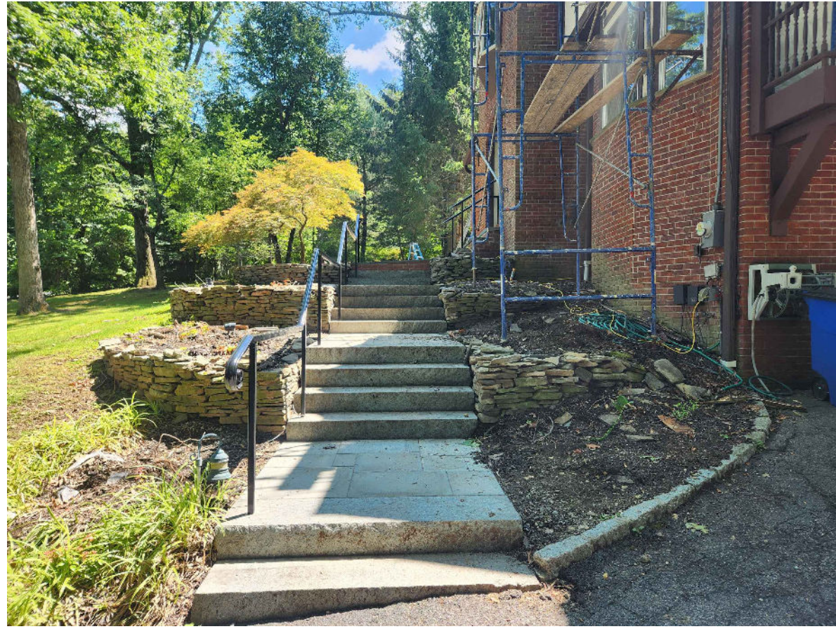
EXISTING RETAINING WALLS AT FRONT OF HOUSE
