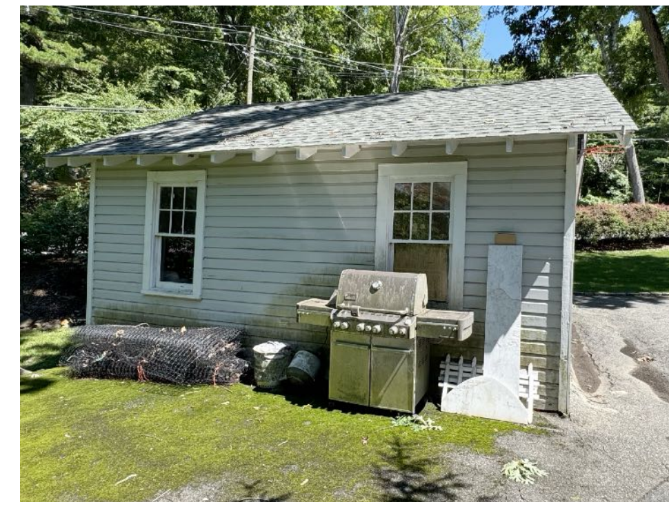
EXISTING NORTH ELEVATION VIEW FROM REAR YARD
